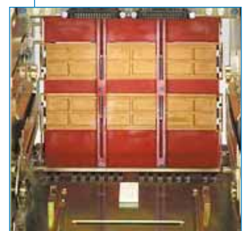
The independently operated and lockable shutter design provides a safe environment when the breaker is removed from the cassette.
